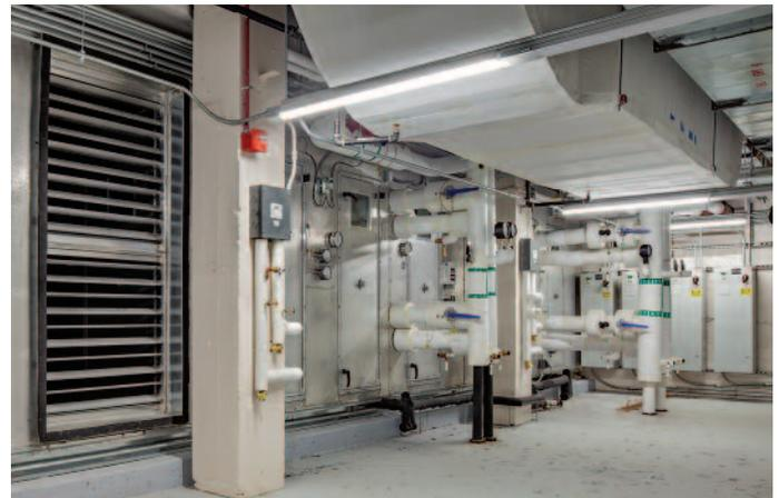
An enlarged sub-basement mechanical room accommodates a custom 30,000 CFM air-handling unit with a remote energy-recovery ventilator (not shown).
