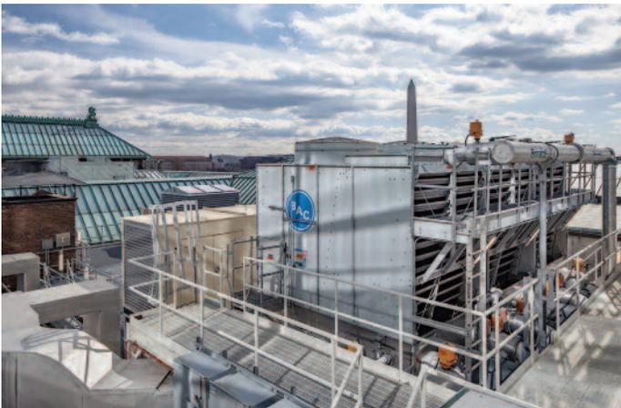
The top elevated platform (left of the roof-mounted cooling tower) accommodates a gas-fired emergency generator, a common outside-air louvered penthouse, and spatial provisions for future air-handling units.
