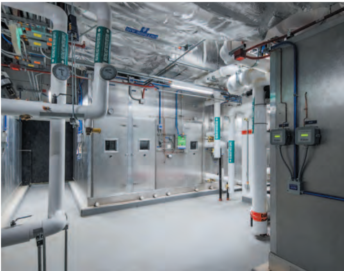
The galleries' sophisticated air-distribution system combines high-performance VAV with dedicated outdoor-air pretreatment, energy recovery, adiabatic humidification, and MERV-15 filtration. This allows precise dehumidification control while minimizing reheat energy through optimized supply-air temperature reset strategies.
